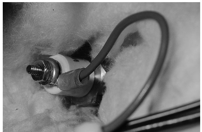
Figure 45. LWCO Probe Installed in Threaded Fitting
